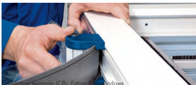
Installation example (CB): Fitting PVC windows
