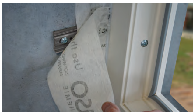
Installation example for ISO-CONNECT VARIO SD „PADS“
