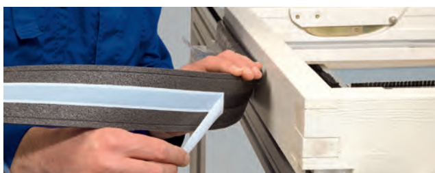
Installation example (1-BT): Fitting wooden windows
