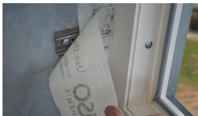
Installation example for ISO-CONNECT VARIO SD „PADS“
