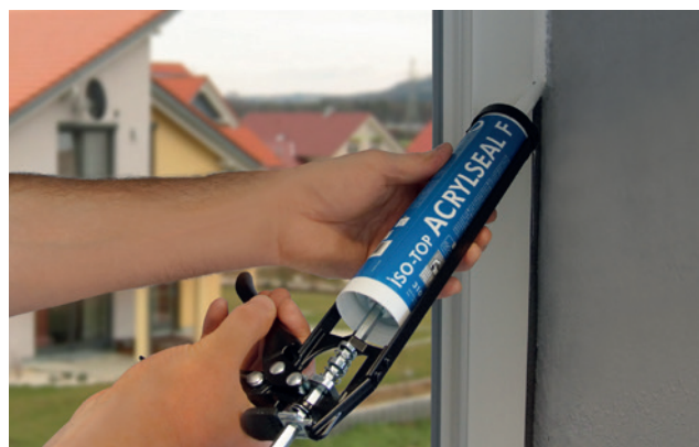
Installation example: ISO-TOP ACRYLSEAL F
