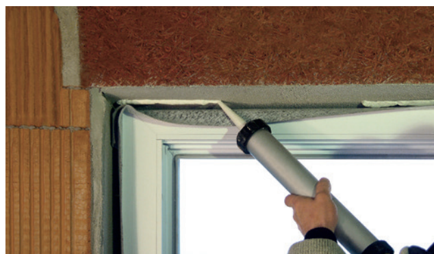
Installation example: ISO-TOP FLEX-ADHESIVE SP
