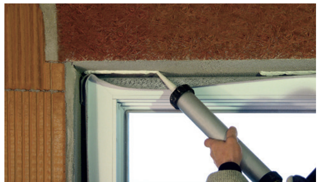
Installation example: ISO-TOP FLEX-ADHESIVE SP
