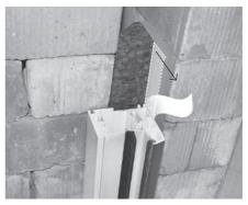
Fix the frame against the stop (check reveal) in such a way that an all-round sealing joint  $\leq 6 \text{ mm}$  is created.
